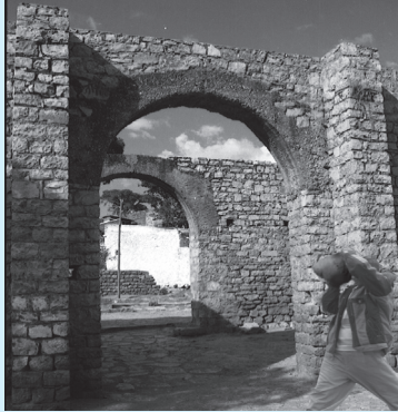
Picture 6.2. The wall of Harar
